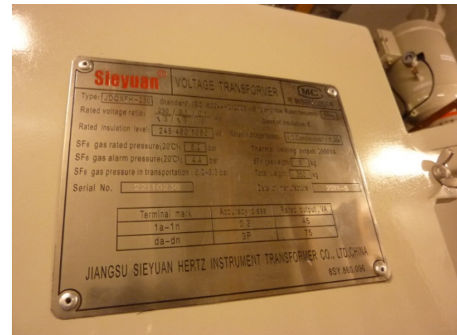
Wound GIS voltage transformers class 0.2
